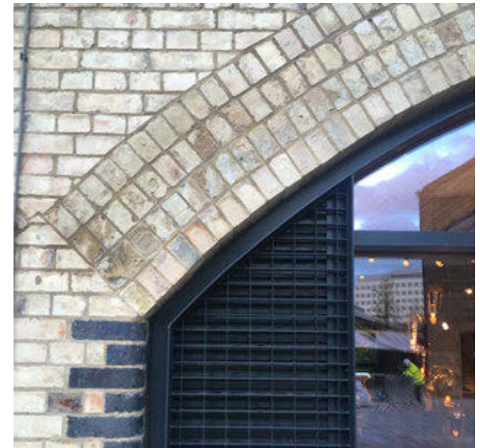
Fig 6.3.125: Examples of fixing to heritage structures
