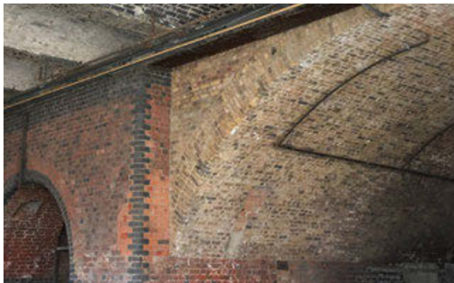
Fig 6.3.121: Existing materiality and patina in Plots 7B, C and D; note the brick detailing around arches and piers
